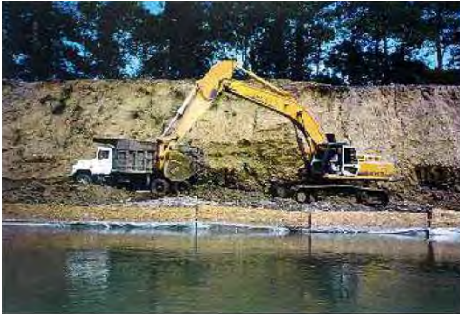
Figure 8.1 Construction platform for major streambank restoration. Source: Inter-Fluve, Inc.
