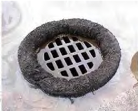
Figure 3.1 At-grade inlet protection method.
