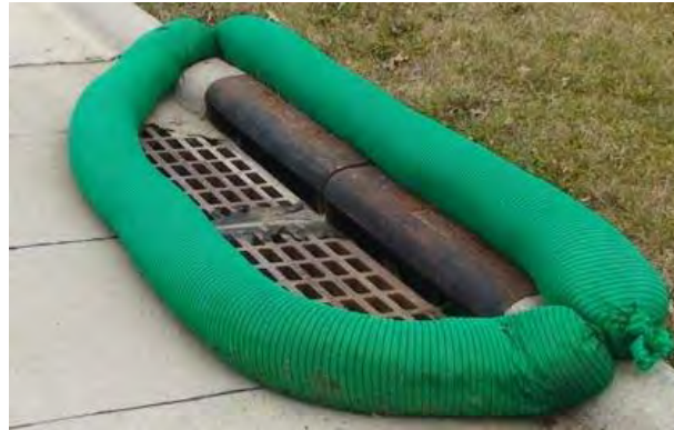
Figure 3.2 Curb inlet protection method.
