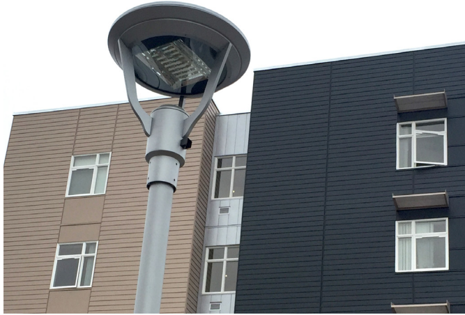
Figure 2: LED site downlight. An array of individual LEDs allow for very directional light.
