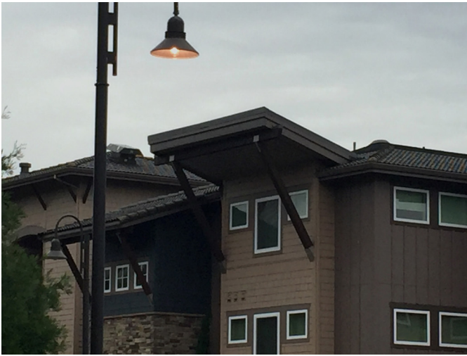
Figure 4: High Pressure Sodium site lighting luminaire.
