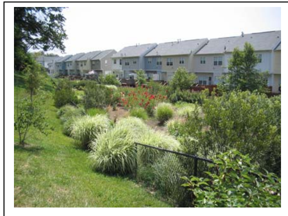
Large rain garden draining a housing complex on Mississippi Avenue, SE, DC in Oxon Creek (Anacostia River)
