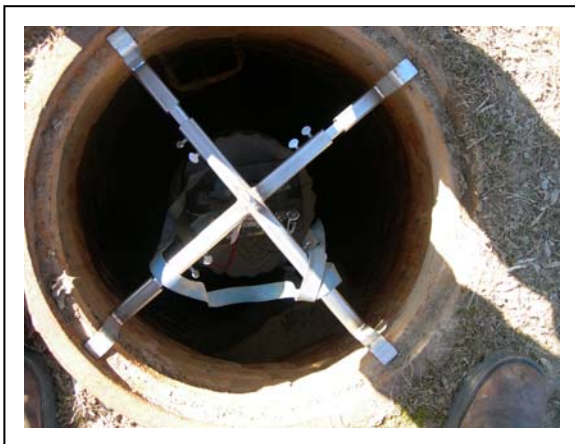
Manhole ISCO Installation for Grab and Composite Sampling.
