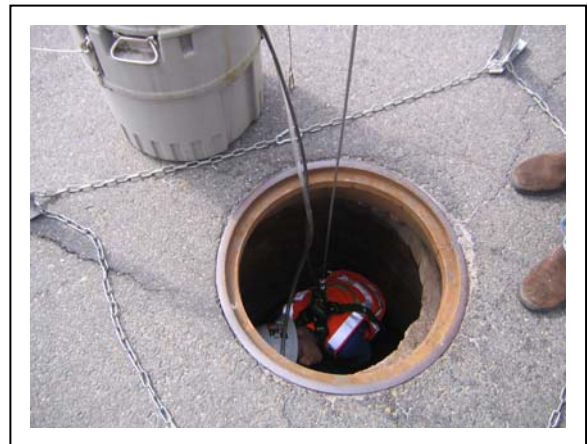
Confined Space ISCO Installation for Grab and Composite Sampling.
