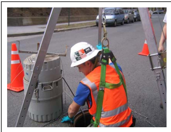
Confined Space ISCO Installation for Grab and Composite Sampling.
