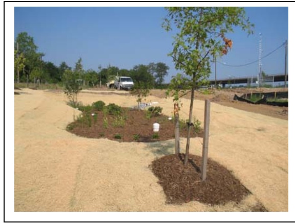
Newly planted rain garden draining Benning Road Bridge, adjacent to Kingman Island, NE, DC
