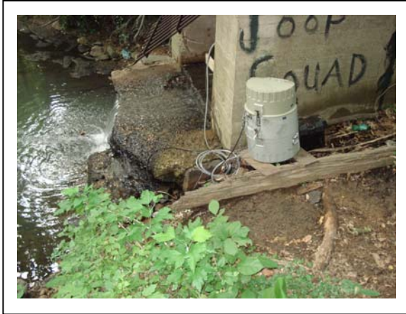
Outfall Installation for Stormwater Composite Sampling.
