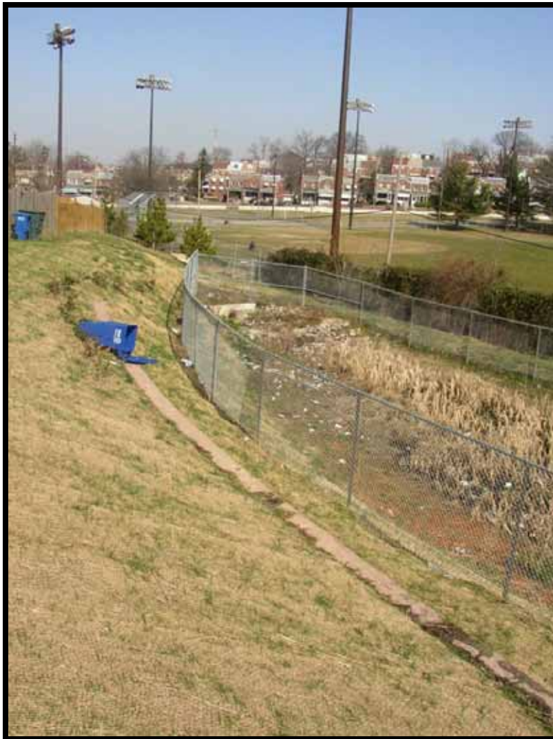
Figure 4.2 Stormwater pond serving a housing subdivision
