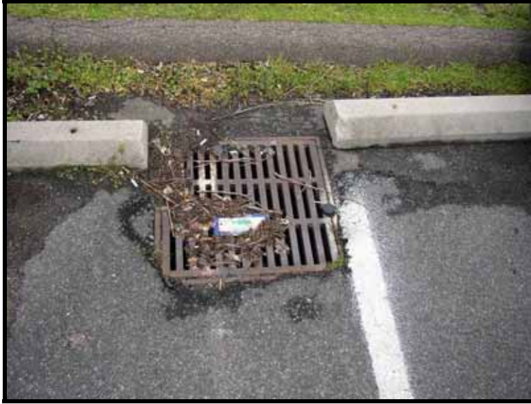
Figure 4.13 DDOE Don't Dump sticker at the James Creek Marina grate
