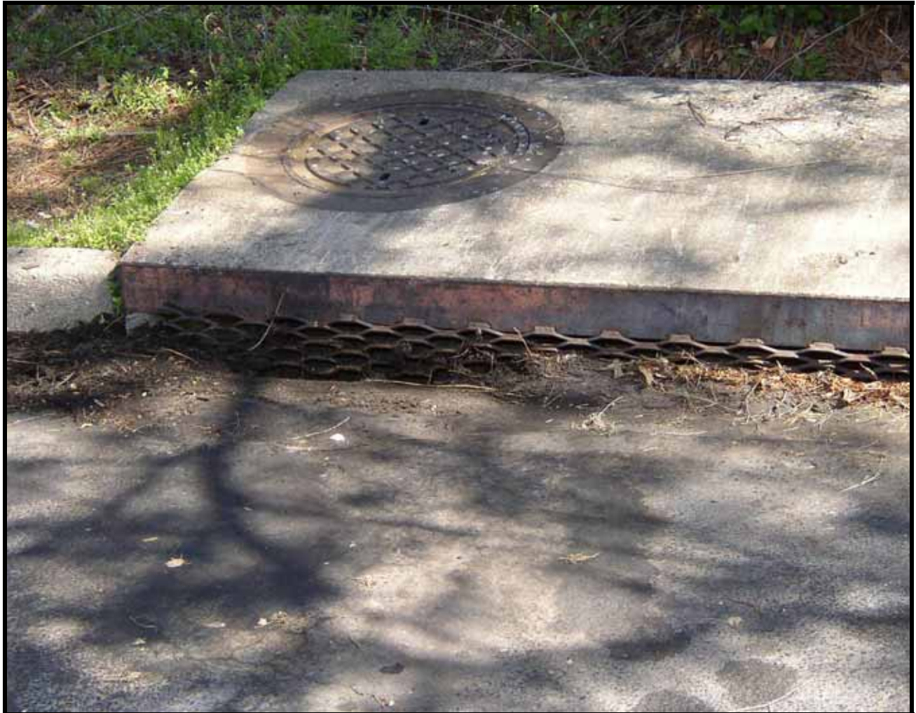
Figure 4.10 Catch basin screen clogged with dirt
