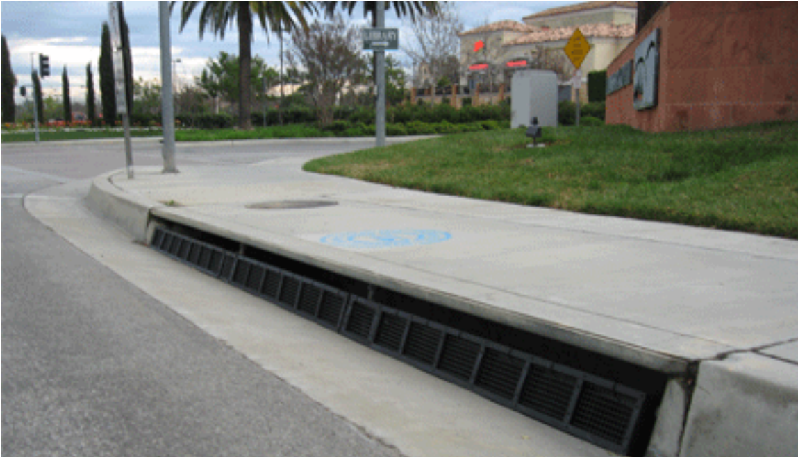
Figure 4.11 Screen grating in Los Angeles
