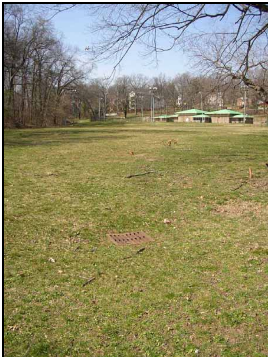
Figure 4.8 Inlet grates used at Langdon Park
