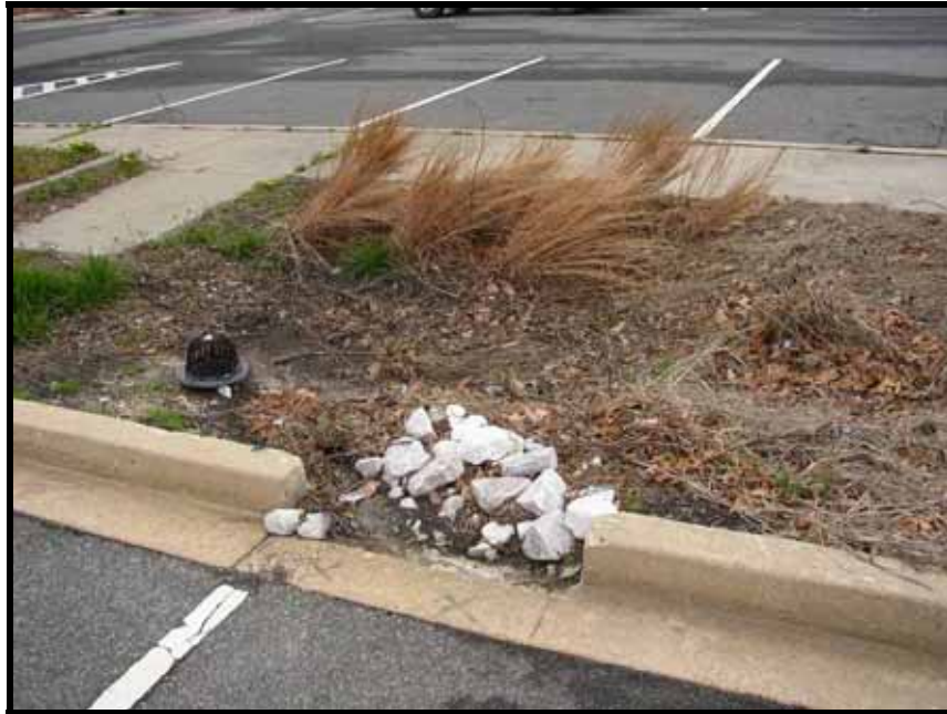
Figure 4.6 Curb cut in the Ely MS4 drainage basin
