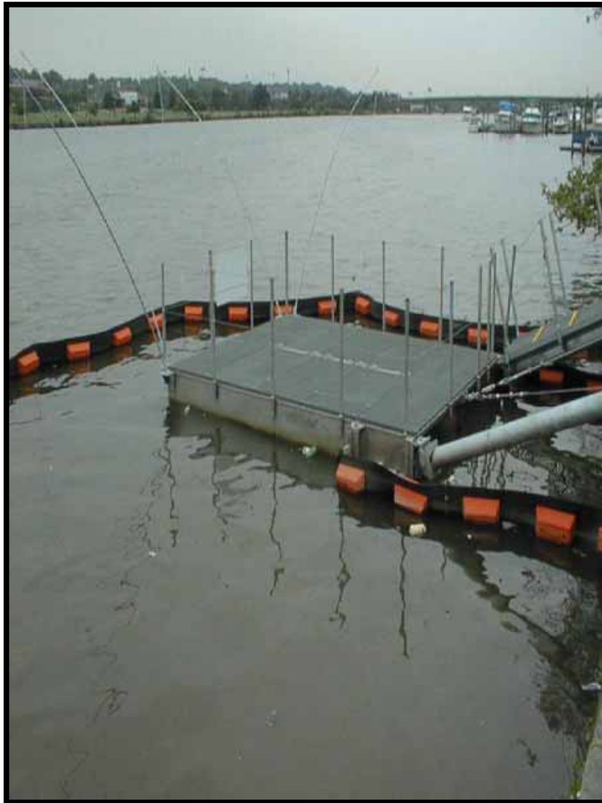
Figure 5.5 WASA Fresh Creek netting system
