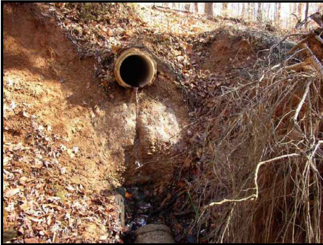
Figure 6.14 Collapsed Storm Sewer Outfall from the Ridge Road Recreation Center
