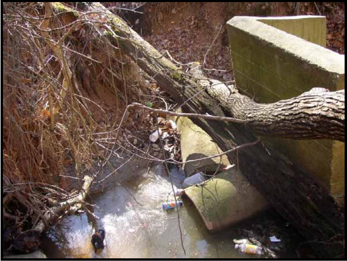
Figure 6.15 Storm Sewer Outfall
