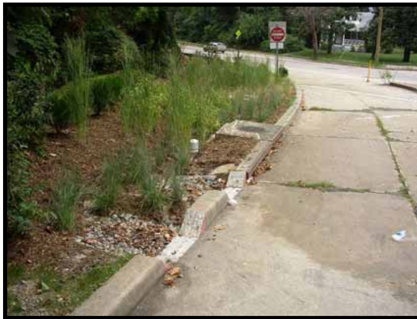
Figure 6.13 Curb cuts and unscreened catch basin
