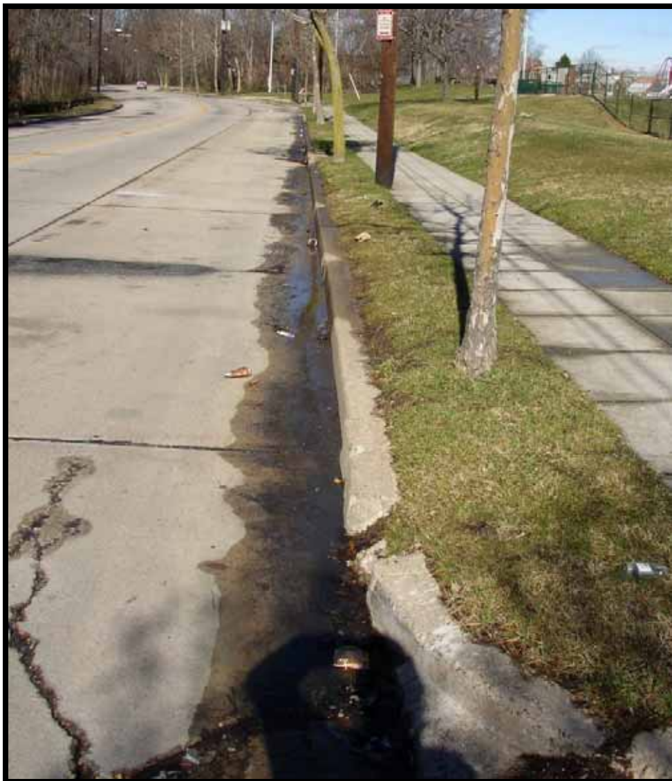
Figure 6.7 Areas Targeted by Street Sweepers and Street Cleaning
