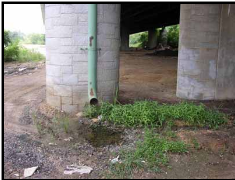
Figure 6.18 Below the elevated portion of the Anacostia Freeway
