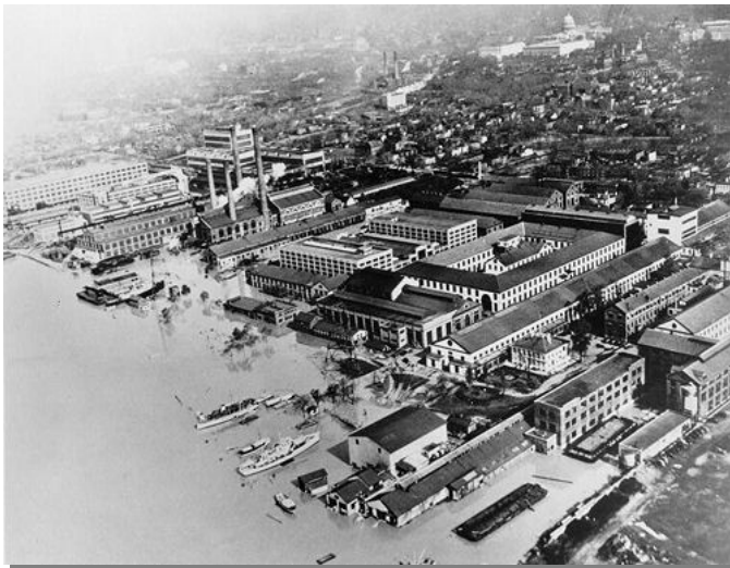
Navy Yard, Washington D.C. during 1936 flooding (Source: Library of Congress)
