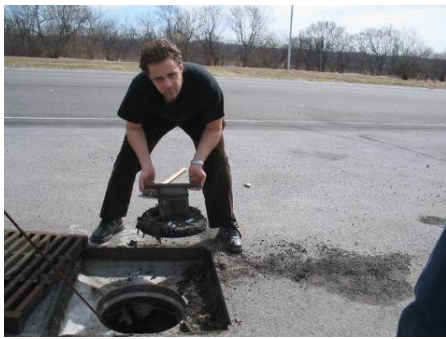
A catch basin insert with collected pollutants
