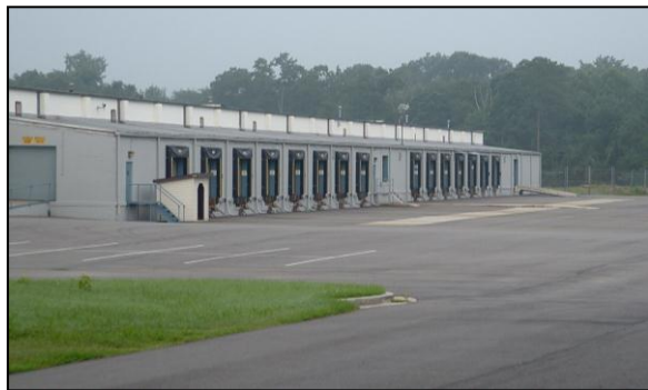
Figure 1: Loading/Unloading Area of Warehouse
