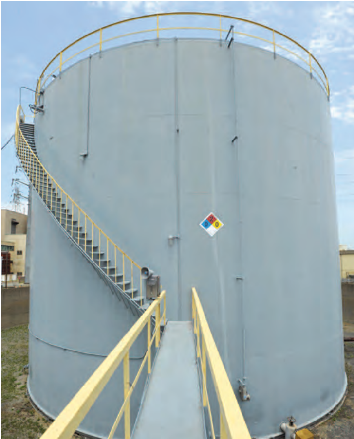
The fuel oil storage tanks that supply the Benning Road Power Plant will be dismantled and removed. Component materials will be properly reused, recycled or disposed of.
