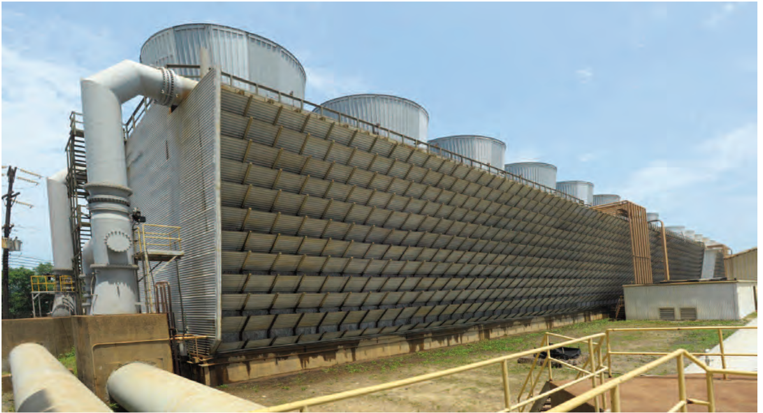
These cooling towers — part of the Benning Road Power Plant — will be dismantled and removed following closure of the plant. PES will arrange for the component materials to be reused, recycled or disposed of according to accepted environmental standards.
