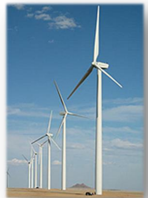
Figure 4-4: These wind turbines near Lamar, Colorado, are part of the 162-MW Colorado Green Wind Farm. Each turbine produces 1.5 megawatts of electricity.
