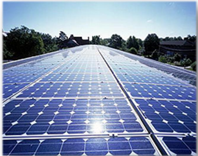
Figure 4-1: Large silicon solar array on the roof of a commercial building
