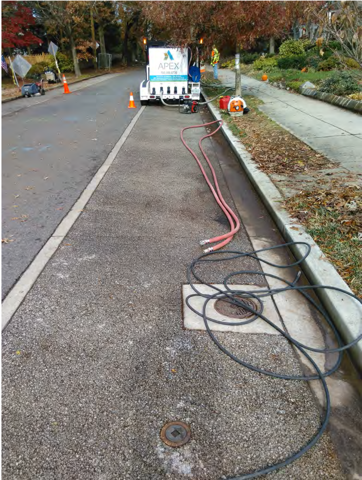
Figure 4-3. Apex Equipment Deployed in Lafayette
