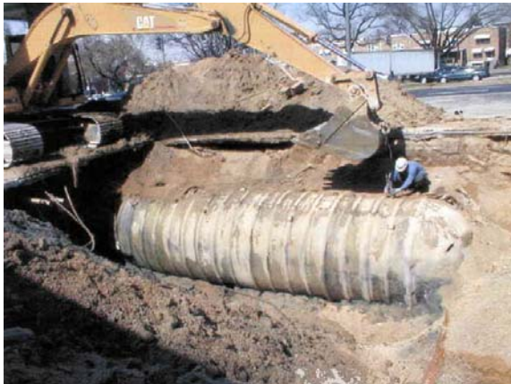
Excavation of UST 1
