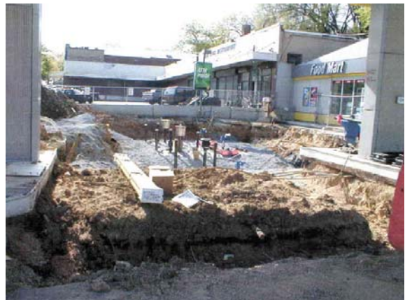
Excavation of Dispenser Area
