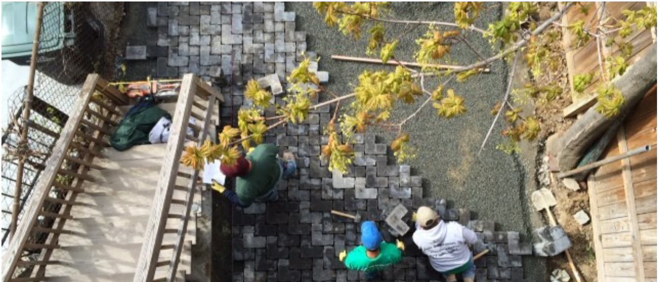
RiverSmart Rebate Pervious Paver Project in Progress
