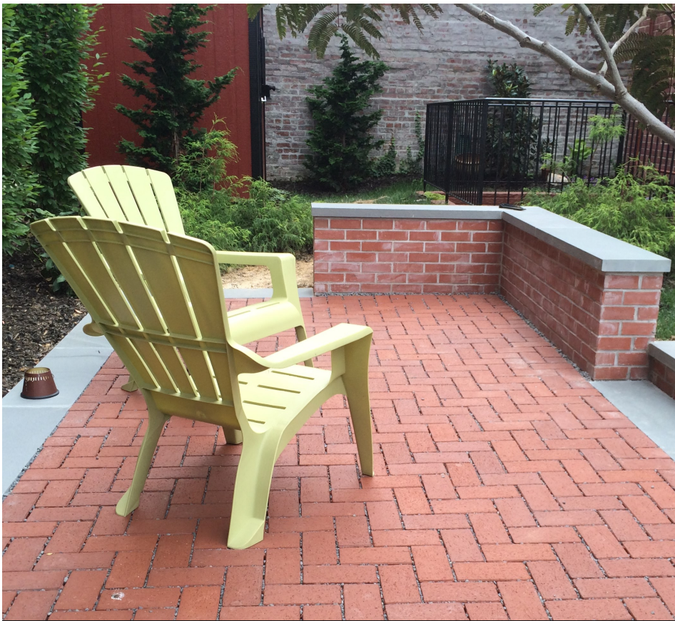
RiverSmart Rebate Pervious Paver Patio
