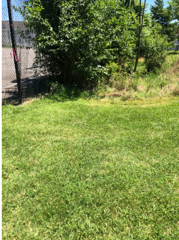
Photo 1: Existing Bioretention Basin
