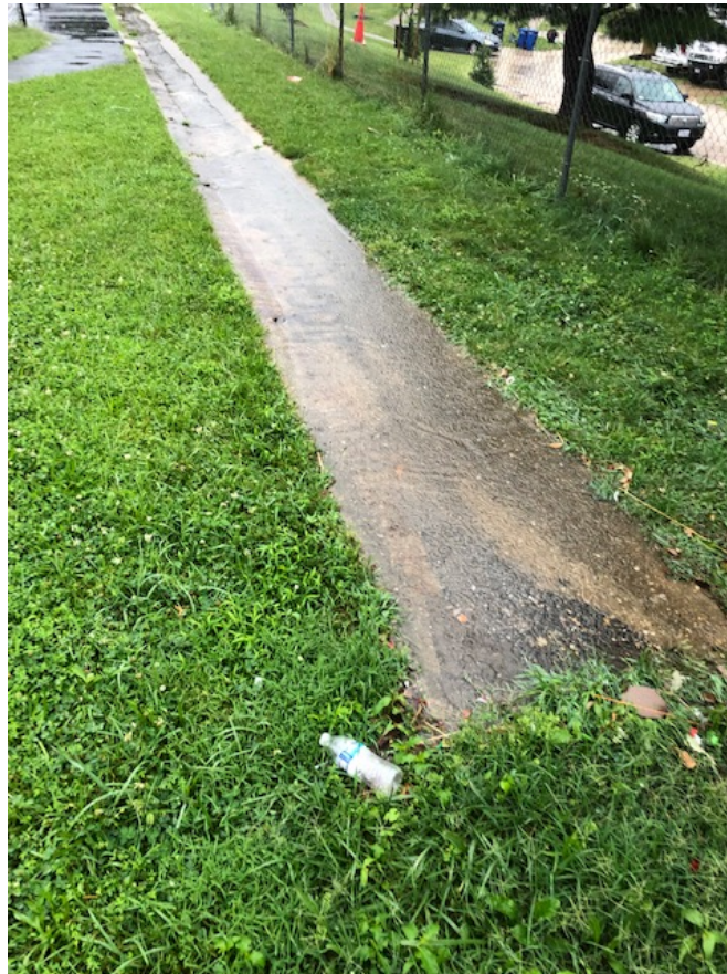
Photo 4: Existing Concrete Ditch
