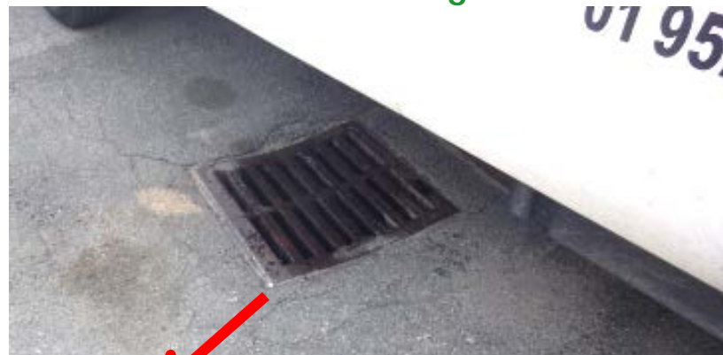
Actively leaking vehicle over storm drain = Illicit Discharge
