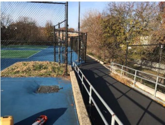
Lower basketball court inlet
