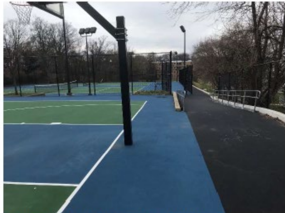
Lower basketball court and inlet
