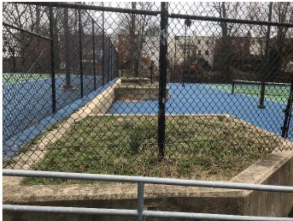
Planter gardens in tennis courts
