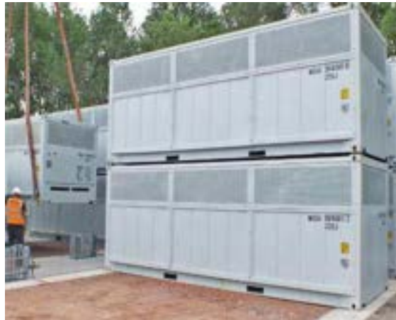
Figure 1: Lithium-ion battery installation
