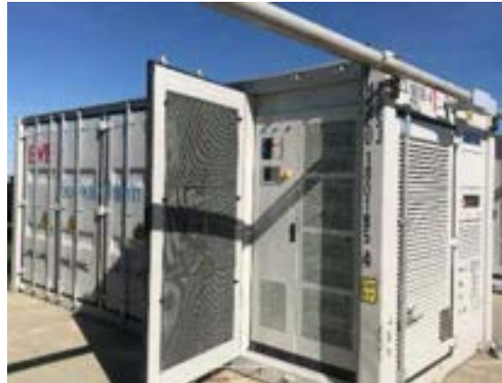
Figure 1: Lithium-ion battery installation
